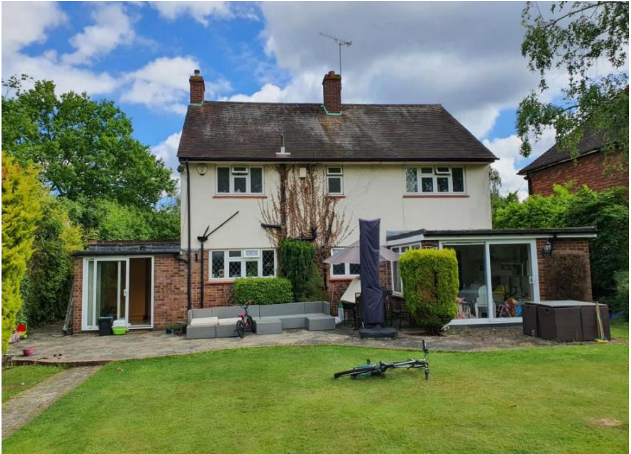
Figure 9: Photo of Rear Elevation
