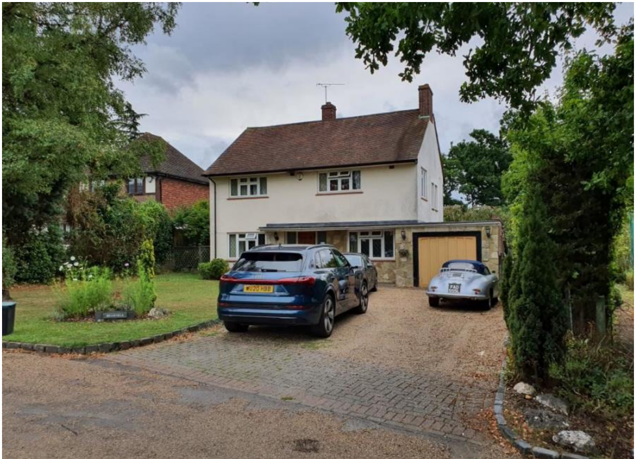
Figure 10: Photo of Front Elevation
